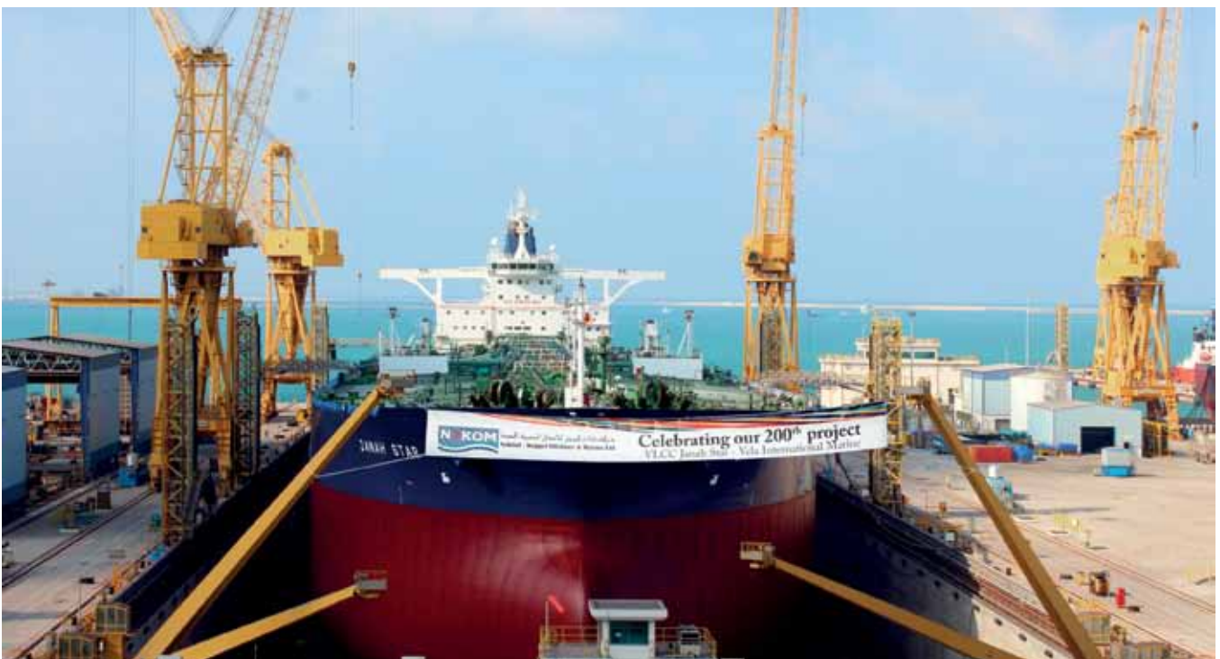
N-KOM completed repair works for the VLCC, M.V. Janah Star, its 200th project since the yard started operations three years ago
