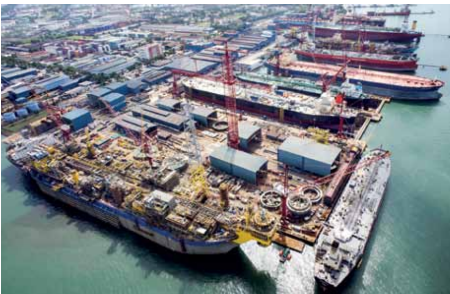
Keppel Shipyard and Keppel Nantong Shipyard secured another five contracts, clear market endorsements of Keppel's extensive expertise and experience in FPSO and FSO conversion, upgrading and repair works
