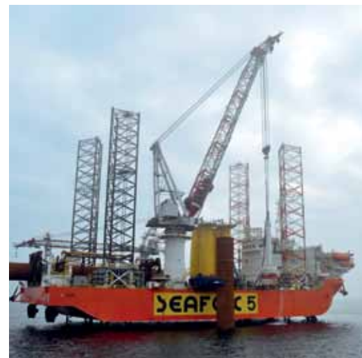
Seafox 5 managed to complete all its foundations installation work and record 980 working days without any time lost to injuries in 2013 despite the challenging weather conditions in the North Sea
